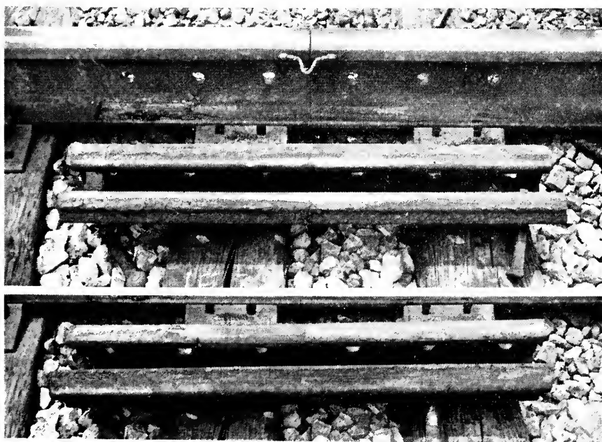
Fig. 17. Section 10. Spray Coat of Texaco TA-2420 after One Year of Service.
